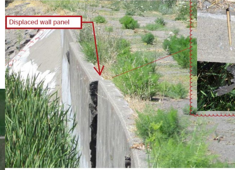
PHOTO 2: Wall 1 Failed Concrete Panel
